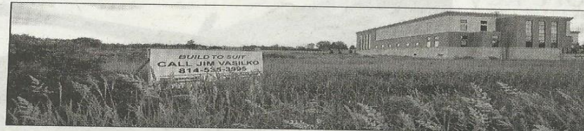
TODD BERKEY/THE TRIBUNE-DEMOCRAT Johnstown Construction Services plans to develop this lot along Eisenhower Boulevard in Richland Township.
